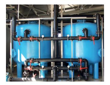
Epoxy Coated Carbon Steel –Inside Neopren Coated Multi Media & Activated Carbon Filters Technical Features
